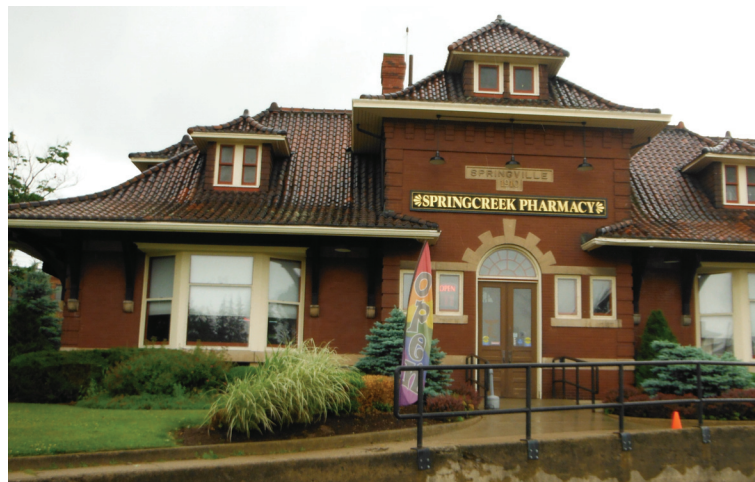
Former Railroad Depot, renovated into a pharmacy, located in the West End Business District
