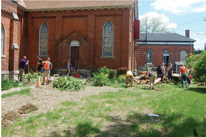
Former Baptist Church, originally constructed in 1869, being renovated into the Springville Center of the Arts
